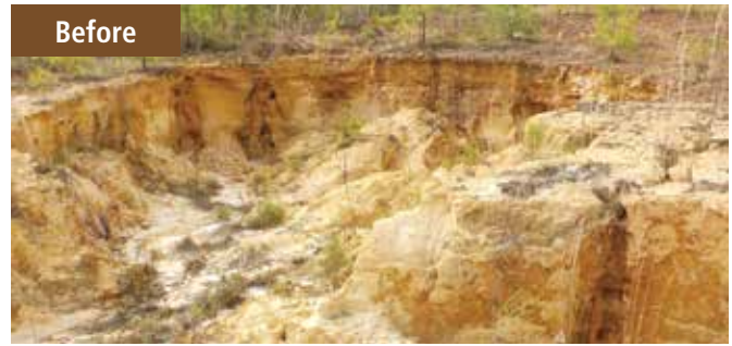
Large gullies formed due to erosion
